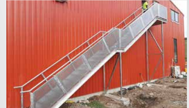
Perforated sheet balustrade & stairs NZ HONEY PROCESSING PLANT
