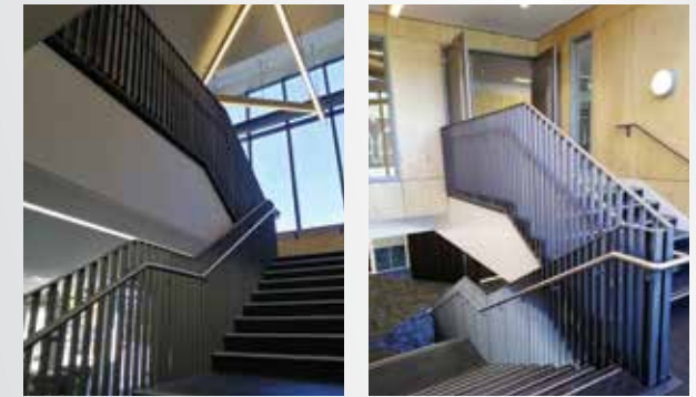
Boys High balustrade & stainless steel handrails MINISTRY OF EDUCATION
