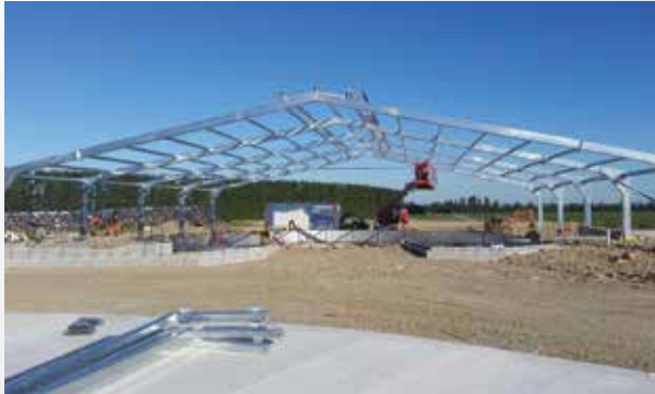
Large structural steel dairy instalment NGĀI TAHU PROPERTIES
